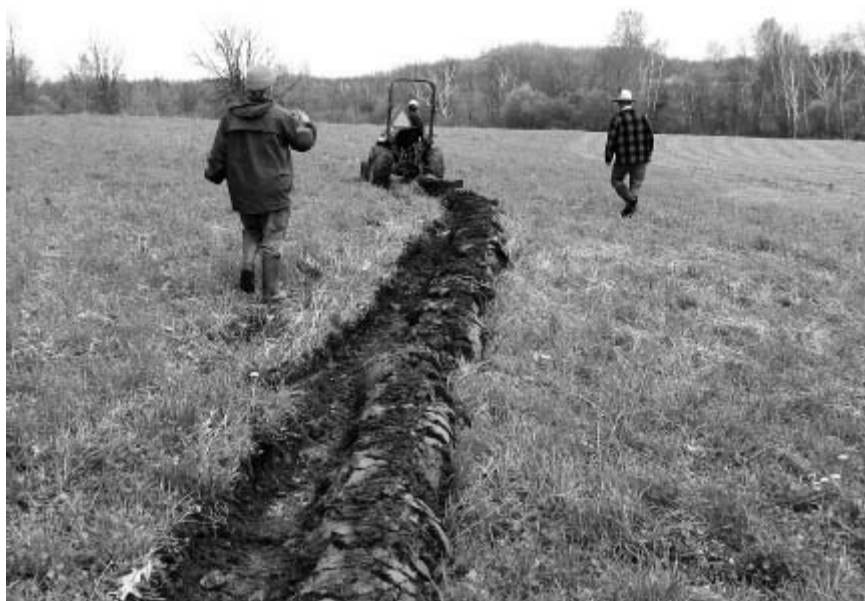
The equipment used is dependent on the size of the site and the soil permeability. It can range from shovels and hoes to bulldozers and excavators.
